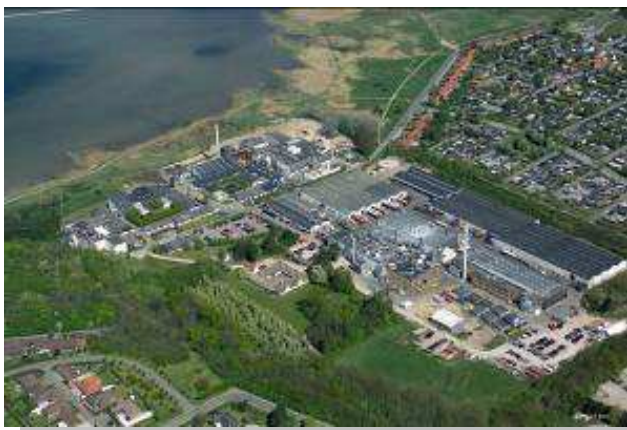
Catalyst plant, Frederikssund, DK
