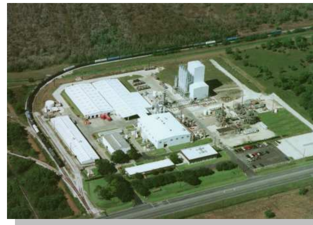
Catalyst plant, Houston, Texas
