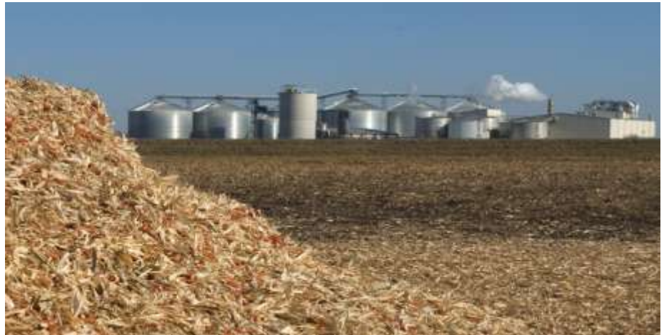
POET Project LIBERTY Integrated Biorefinery Near Emmetsburg, IA
