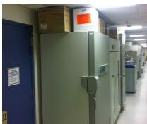
Each ULT freezer occupies 20-30 ft<sup>2</sup> of valuable space. Due to space constraints in labs, numerous ULT freezers are stored in hallways (figure 14). Most hallways are not designed not effectively remove heat generated from ULT freezers; therefore, ambient temperatures can be as high as 90°F (32°C). Operating ULT freezers at these ambient temperatures increases energy consumption by as much as 24% and increases the risk for a ULT freezer to fail, which puts samples at risk.
