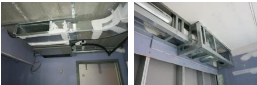
Figure 8. HVAC placement in apartment ceilings. Heat pump above entryway, no drop ceiling installed yet (L); inline fan boxed into soffit (R).
