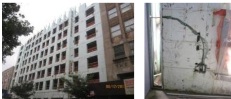
Figure 7. Insulated concrete form exterior wall construction (L); typical channel through exterior wall for electrical (R)
