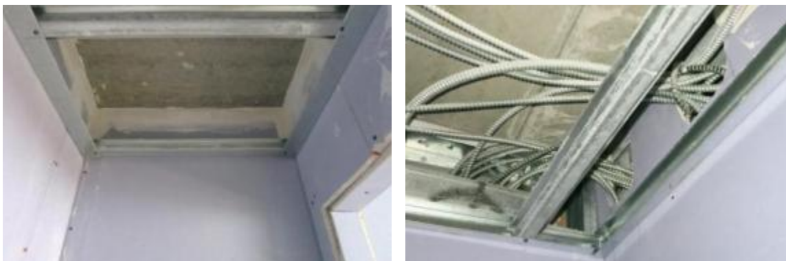
Figure 10. Effective drywall layering in ceiling cavity (L); compromised ceiling cavity air barrier (R)
