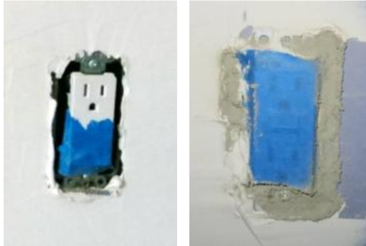
Figure 16. Typical electrical outlet before sealing; another outlet after sealing
