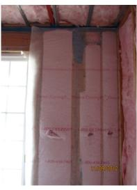
Figure 6. Exterior wall air sealing and insulation used at CV and SH
