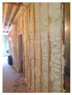
Figure 11. Demising wall air sealing at HV
