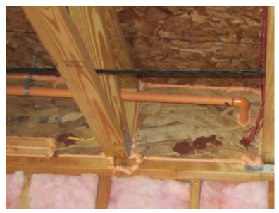
Figure 8. Air sealed plywood smoke curtain used at demising wall of CV
