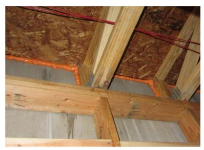
Figure 9. Air sealed sheetrock smoke curtain used at demising wall of SH
