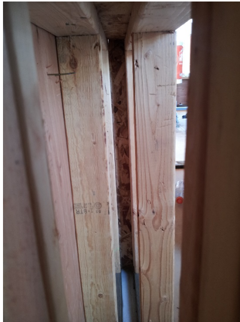
Figure 10. Lateral double-stud wall cavity view
