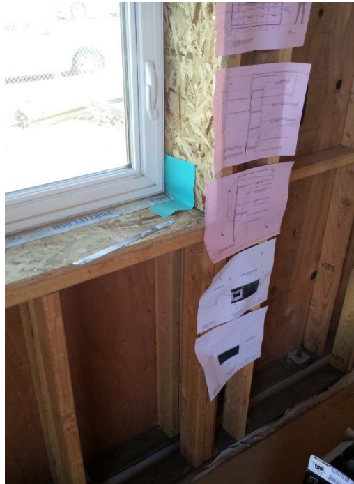
Figure 11. OSB framing detail at window
