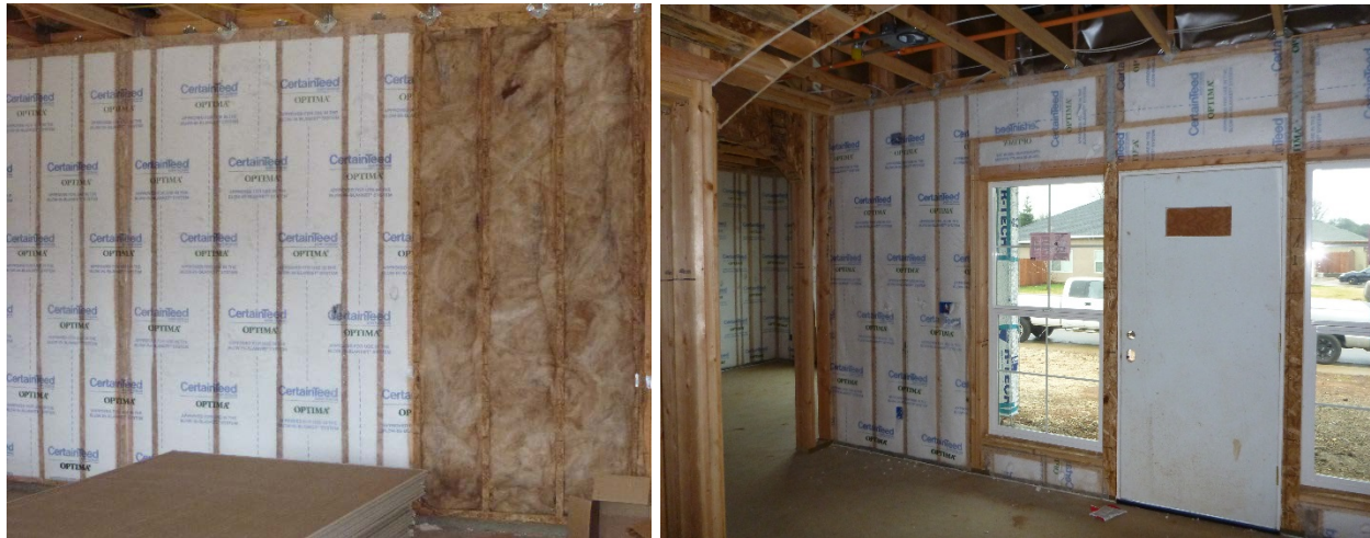
Conservative use of studs and high quality insulation
