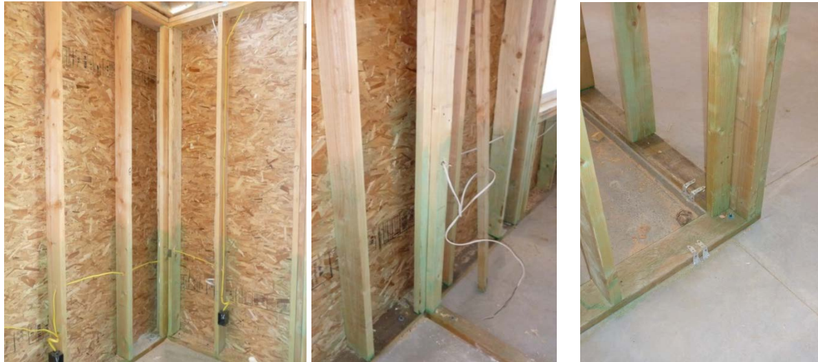
Intersecting exterior wall
