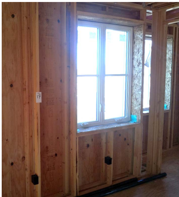
Figure 12. OSB board window perimeter connection
