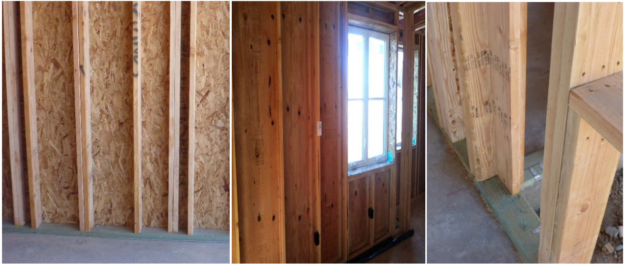
Use of 2 × 4 studs to minimize thermal bridging
