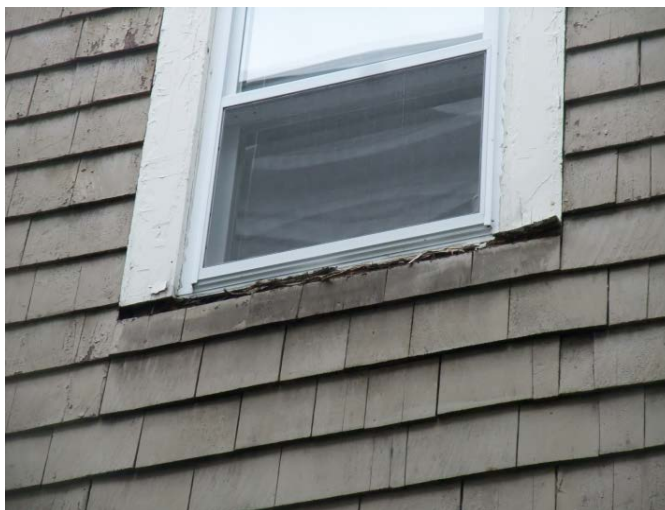
Figure 5. Failed window sill with replacement window installed
