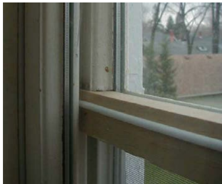
Figure 30. Window sash modification
