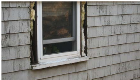
Figure 18. Abandoned sash weight and insulation installation
