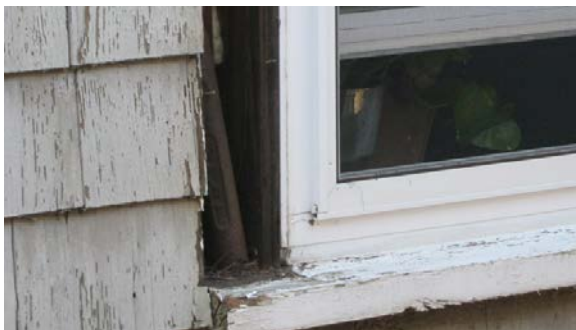
Figure 17. Sash weight pockets
