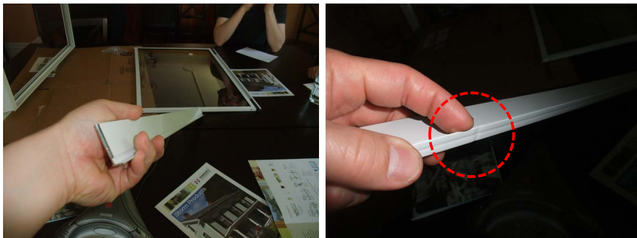
Figure 36. Exterior aluminum storm windows, showing weep channel
