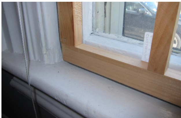
Figure 26. Installed interior removable storm window
