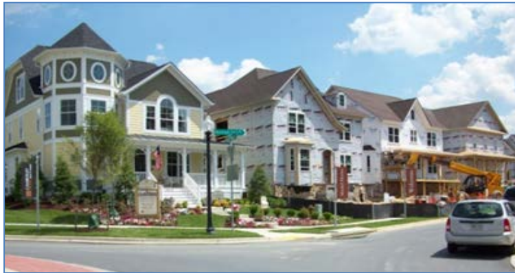
Figure 11. Three additional houses built using NCTH features
