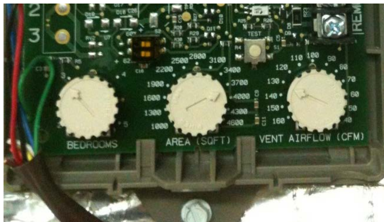
Figure 17. Ventilation control settings.
