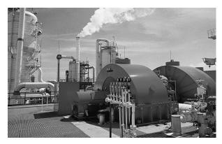
**Power Around the Clock** This turbine generator works fine outdoors at a geothermal project in California's Imperial Valley. Geothermal power plants provide baseload power, so these turbine generators operate 24 hours a day. *(Photo courtesy of Geothermal Education Office, Tiburon, CA)*
