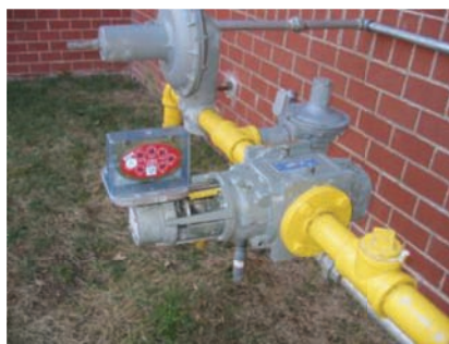
Gas Rotary Flow Meter
