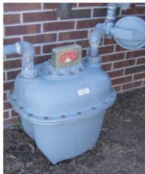
Natural Gas Diaphragm Meter
