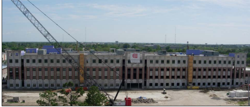
Figure A5. The 400,000 ft 2 MARFORRES HQ building (photo taken April 12, 2010)
