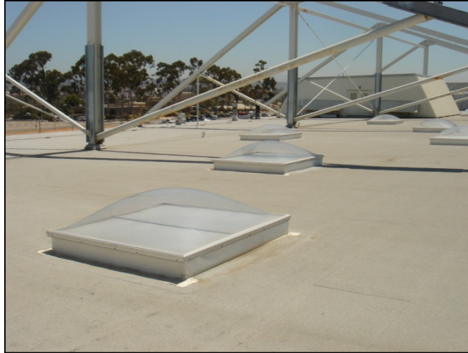
Figure A3. Daylighting on a hangar at Miramar
