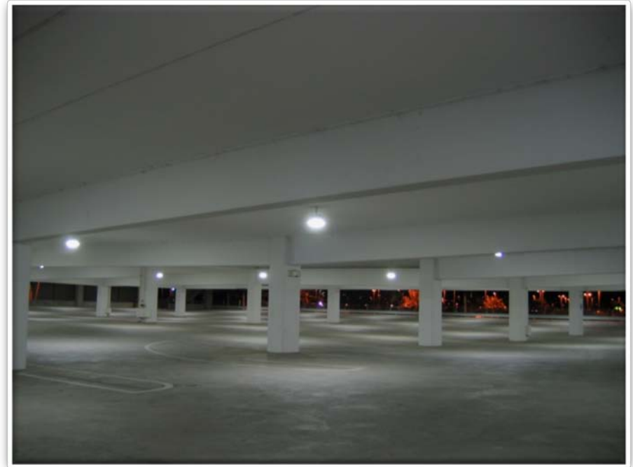
Ceiling and columns painted white Arizona State University, Tempe, AZ
