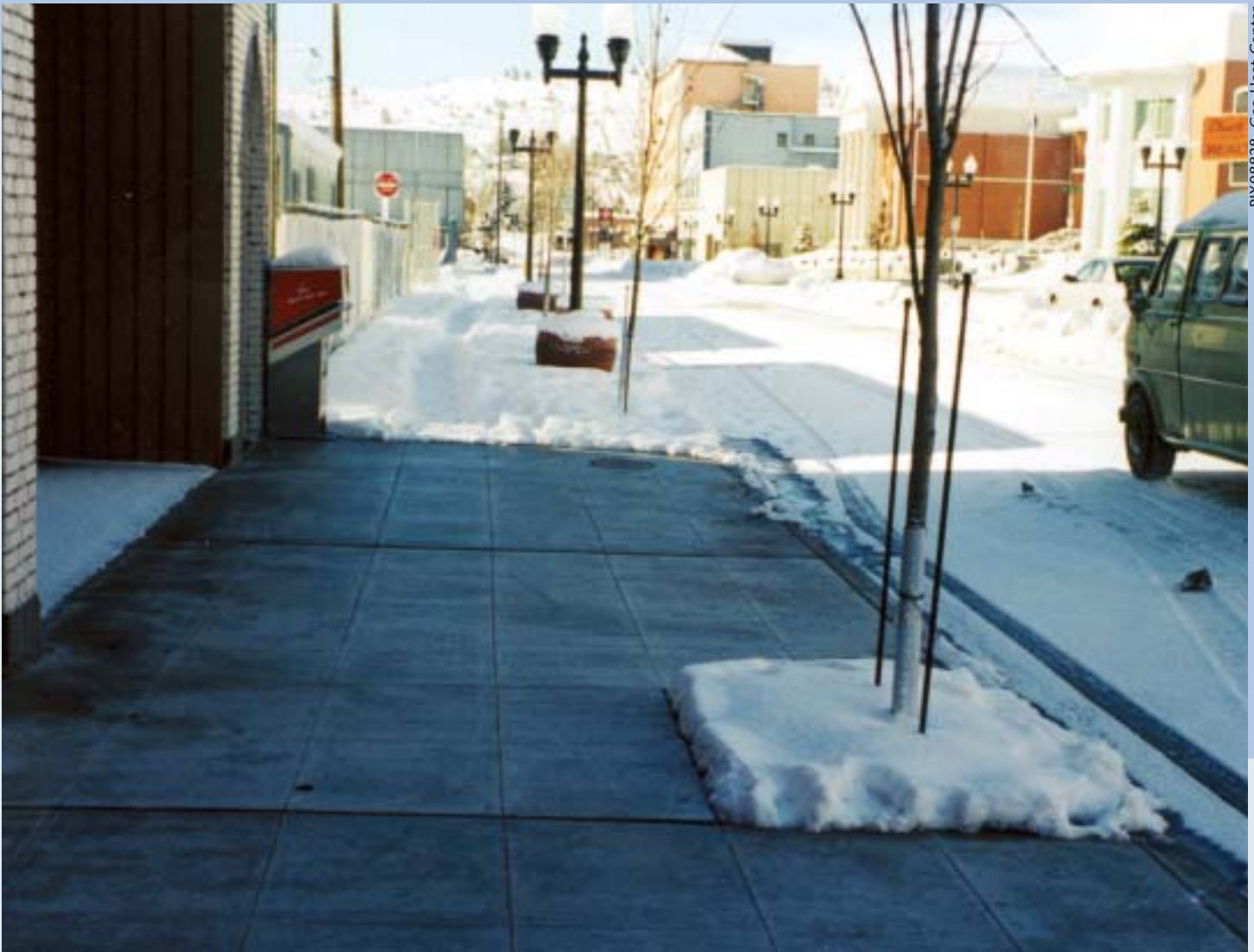
DOE partnered with Klamath Falls, Oregon, on this district heating project. Circulating geothermally heated water under the pavement keeps sidewalks clear of snow and ice.
