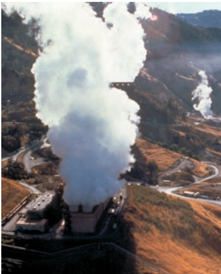
A view of several geothermal power plants at The Geysers, northern California (showing water-vapor emissions during normal cooling operation).
