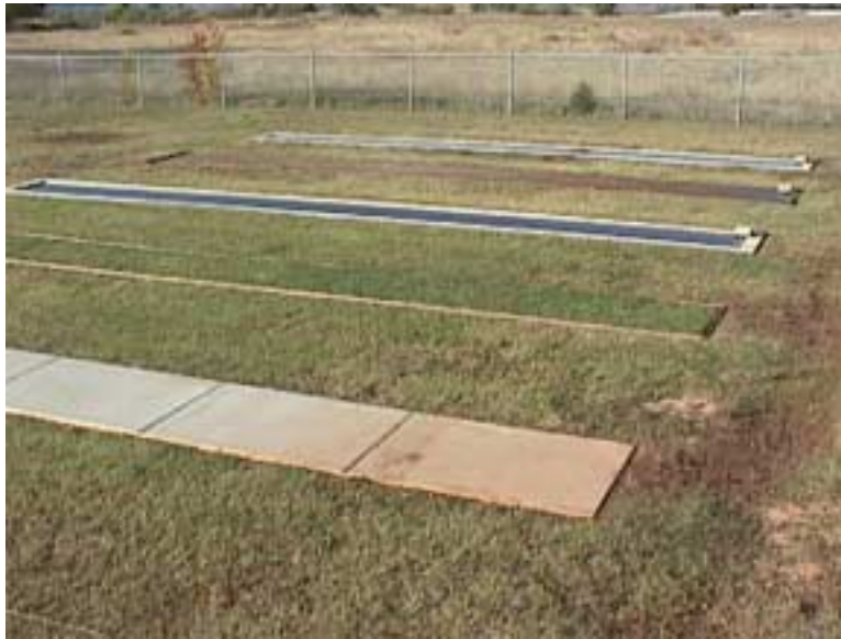
Figure 1. Five Shallow Heat Exchanger Systems.
