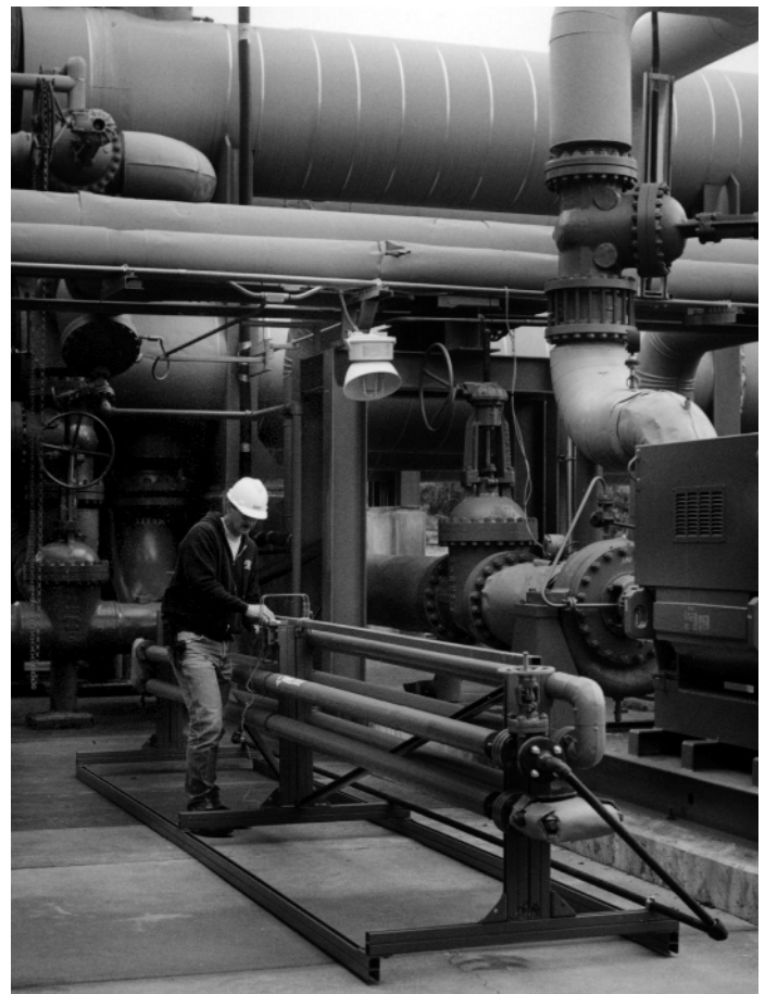
Coating test rig installed at the Mammoth Lakes Power Plant.
