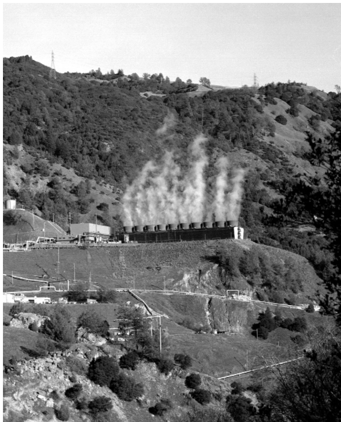
A power plant at The Geysers.
