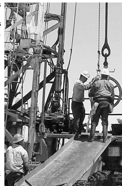
Figure 2: Rigging up to begin borehole televiewer logging in well 82-5.
