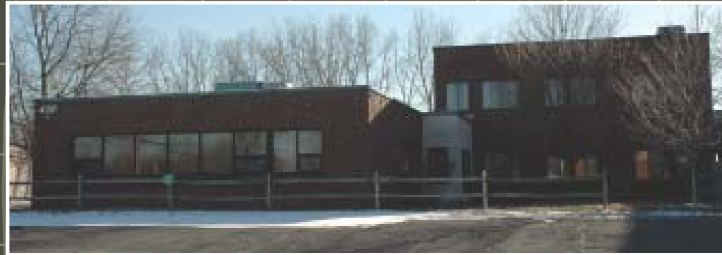
H2 Pump Facilities
