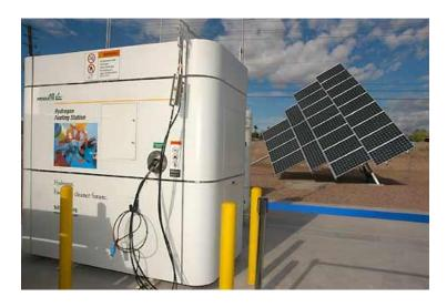
This hydrogen station in Las Vegas, Nevada, uses a solar array to produce hydrogen via electrolysis. The station serves hydrogen vehicles used by the Las Vegas Valley Water Department, and the hydrogen storage is provided by Air Products.
