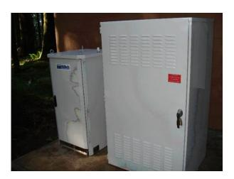
This IdaTech PEM fuel cell system provides back-up power to the Oregon State Police emergency response transmitters. The fuel cell replaces a diesel generator.
