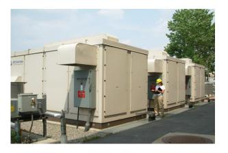
The Hunts Point Waste Water Treatment Plant, in the Bronx, New York, uses three 200 kW units from UTC Power that operate in parallel with the grid.
