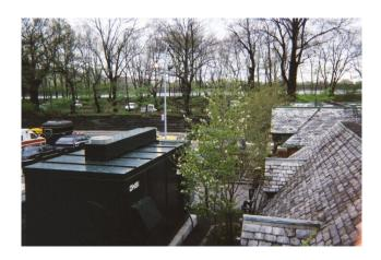
New York Police Department in Central Park uses a 200 kW phosphoric acid fuel cell from UTC Power that operates independently from the grid. During a major city-wide power outage in 2003, the station was unaware of the situation because the fuel cell continued to supply electricity to the building.
