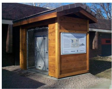
This 5 kW Plug Power PEM fuel cell was installed as a demonstration unit at the Washington Park Fire Station, in Denver, Colorado. The fuel cell provided electricity and heat to run the station's computers, lights and garage door. There are plans to replace the unit with future production models.
