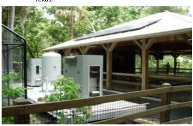
A 5 kW photovoltaic array on the roof of this pavilion runs an electrolyzer that generates hydrogen fuel for a Hydrogenics PEM fuel cell at Homosassa Wildlife Park, Homosassa, Florida.
