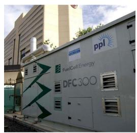
The Sheraton Hotel in Edison, New Jersey uses a 250 kW molten carbonate fuel cell from FuelCell Energy. The fuel cell provides 25% of the hotel's electric and hot water needs.
