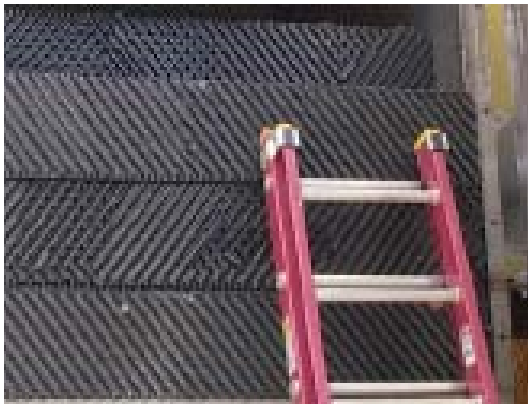
Cross-flow media in the biotrickling module
