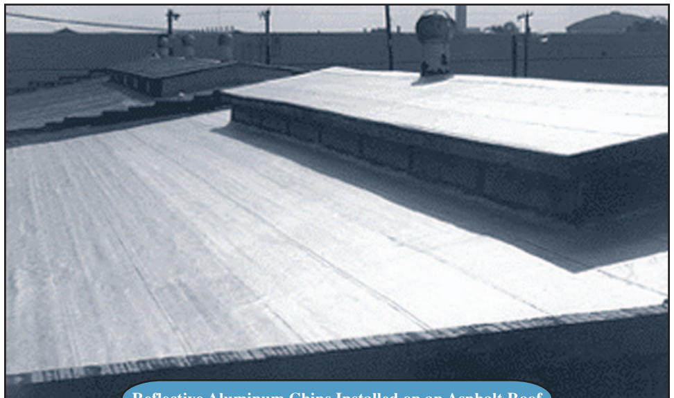
Reflective Aluminum Chips Installed on an Asphalt Roof
