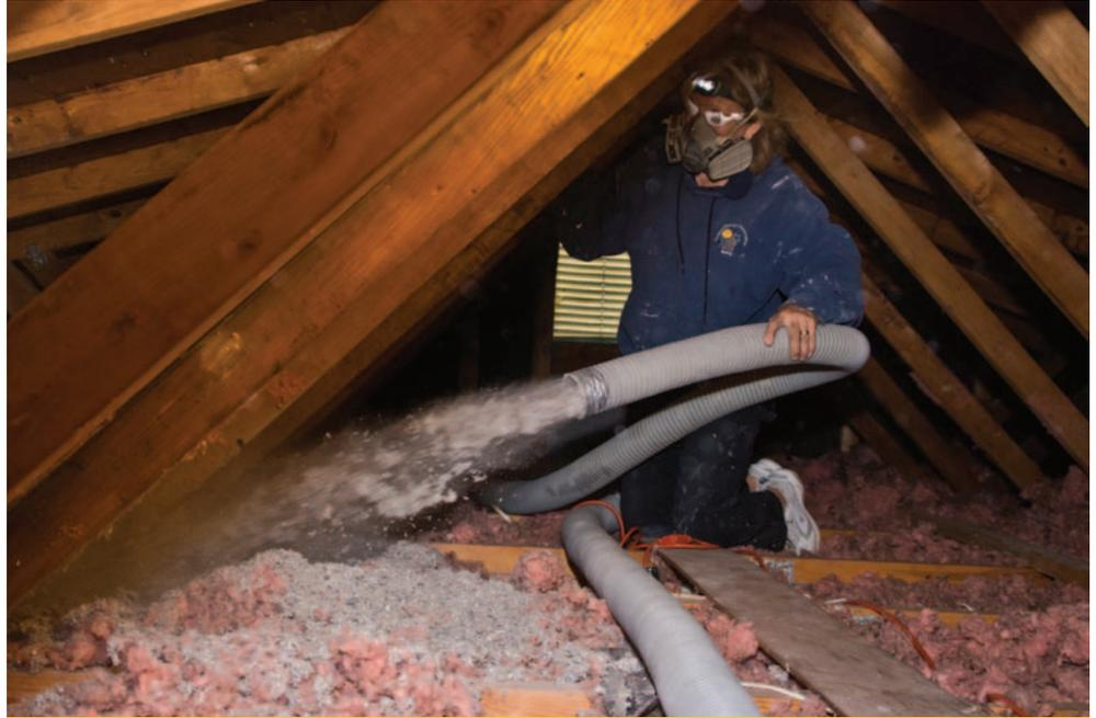
A weatherization crew member blasts insulation into the attic and wall cavities of a client's home.
