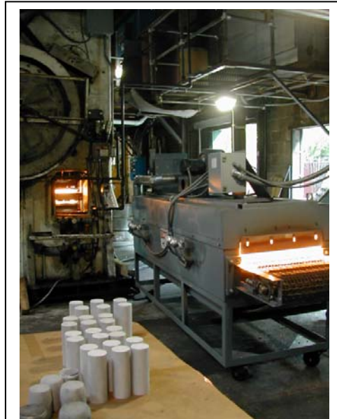
Figure 1: the Advanced Heating System used for preheating aluminum billets at Queen City Forging Company, Cincinnati, OH
