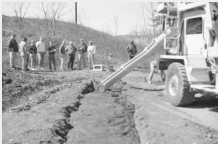
Field testing of controlled low strength material containing foundry sand.
