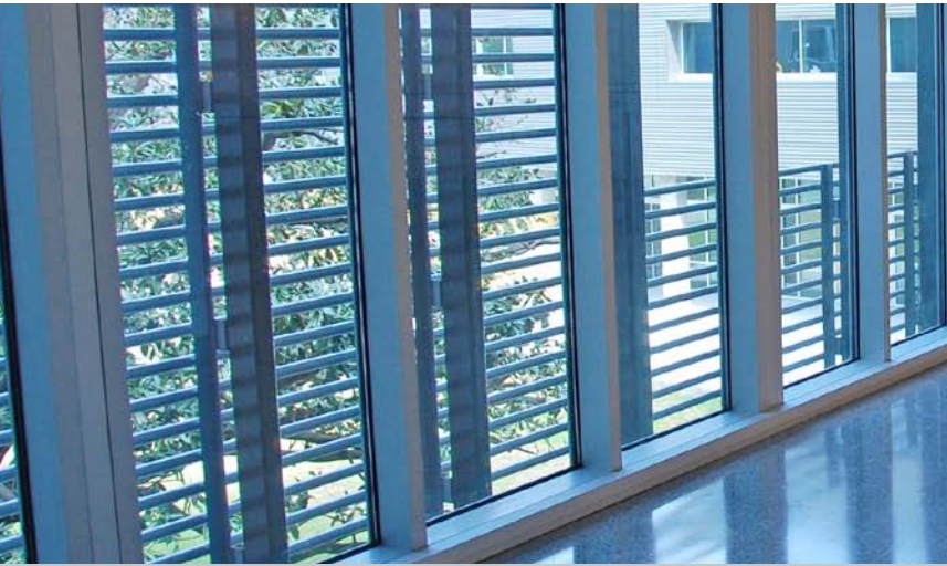
Good daylighting, as shown in the second-floor hallway at L.B. Landry High School, can have numerous benefits, including improving student performance on math and reading tests. Photo by Joe Ryan, NREL/PIX 19720
