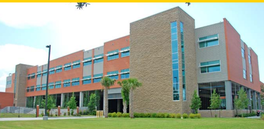
Lake Area High School's design team addressed the deep flooding experienced during Hurricane Katrina by designing the school to be above ground with a ground-level parking garage. Photo by Joe Ryan, NREL/PIX 19646
