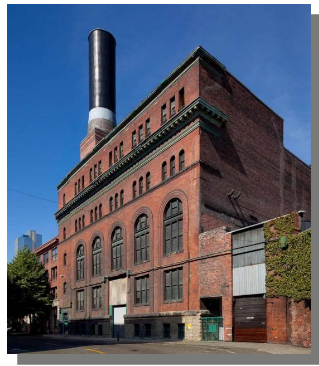
Seattle Steam's historic plant, where the advanced turbine will be installed
