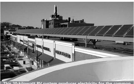
This 20-kilowatt PV system produces electricity for the common areas of a shopping center in Cambridge, Massachusetts.
