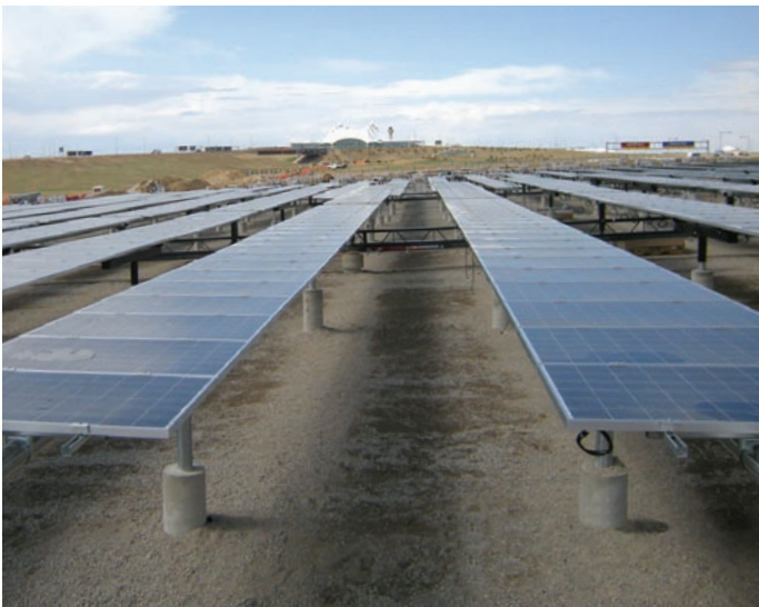
Denver, a Solar America City, installed a 2-megawatt PV system at Denver International Airport.
