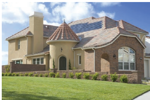
Shea Homes included BIPV as standard equipment on homes in this California development.
