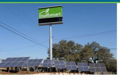
This 11.28-kW PV system was built in 2010 for a net-zero solar model home that was certified as a Level 3 Solar Home by Build San Antonio Green. Photo from Solar San Antonio, NREL/PIX 19479
