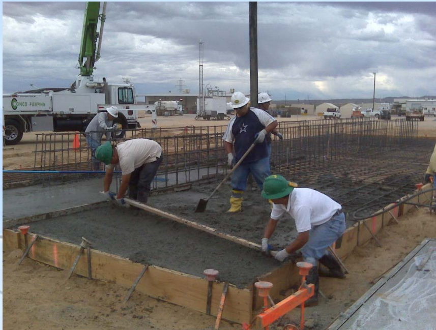
Pouring concrete for the base of the jig
