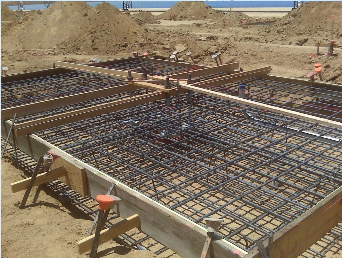
Setting the anchor bolts for the drive pylon
