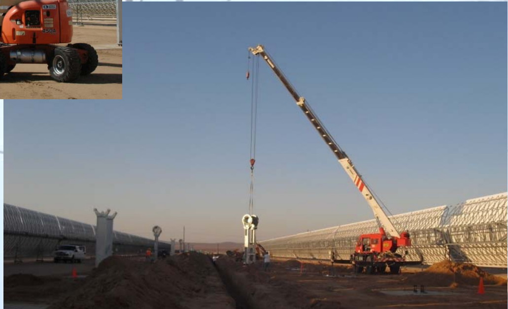
Pylon Erection
