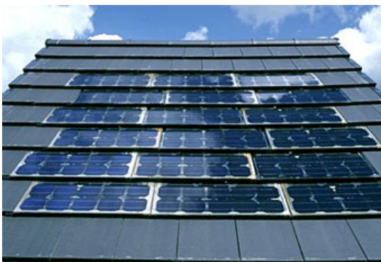
Figure 10: Solar roof tiles demonstrating the potential for large automated snap-together PV.
