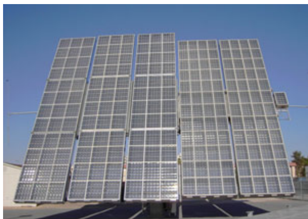
Fig. 2 Three 16" MegaModules and two 21" MegaModules ready for comparison testing at University of Nevada Las Vegas with small multijunction module attached to center right portion of last MegaModule for reliability testing.
