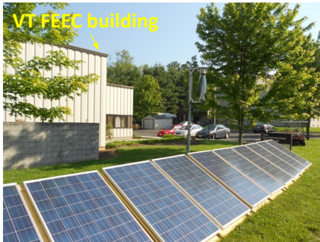
Front view of PV panels
