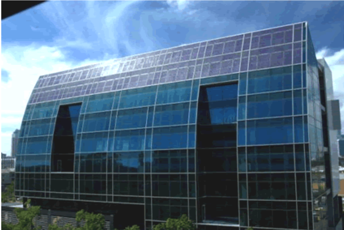
Photo: BIPV Facade, Melbourne University Private (photo: S.Troman)
