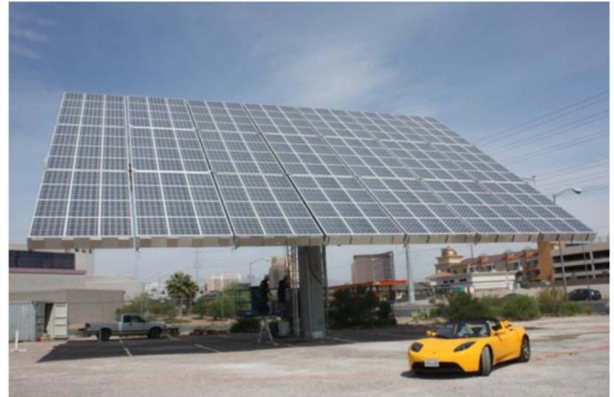
60kW Multijunction Solar Cell (27% AC Efficiency)
