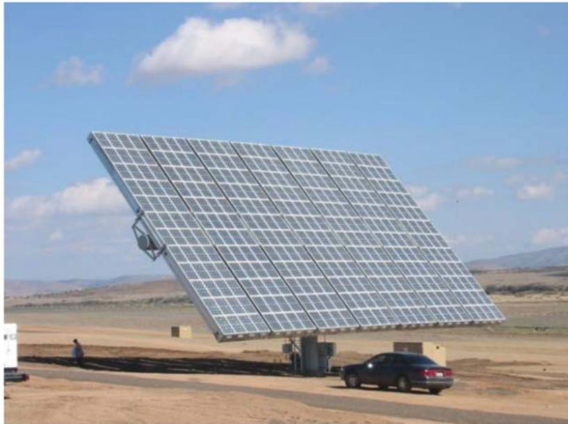
35kW Silicon Cell (16% AC Efficiency)
