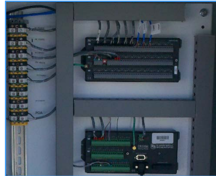
Clean installation; good wire management; rated devices.
