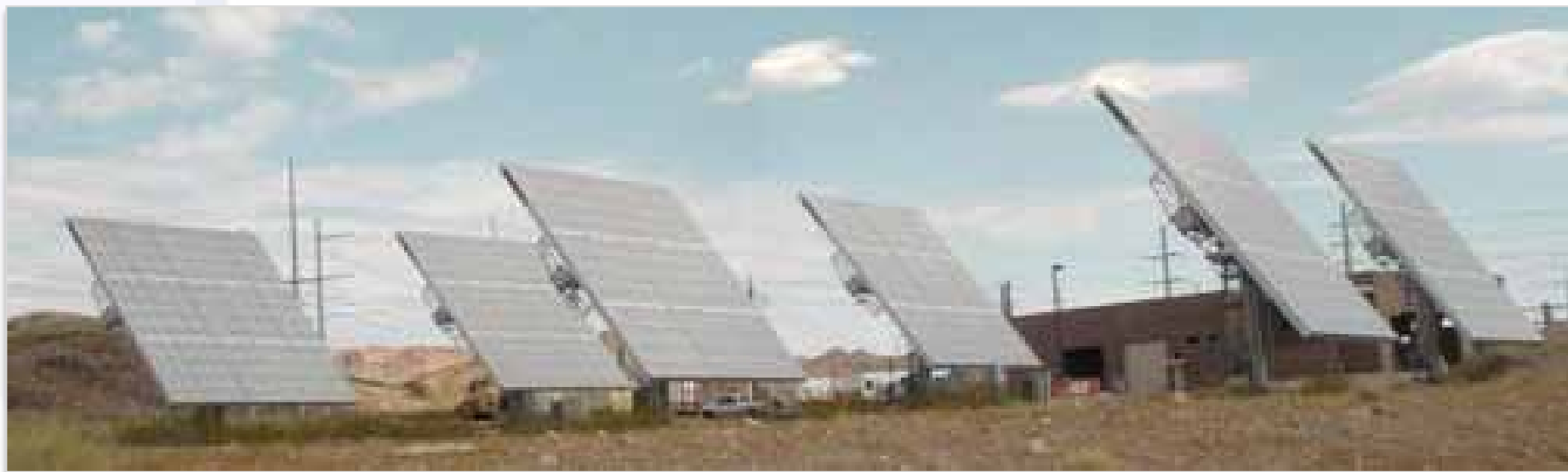
RIVER MOUNTAIN WATER TREATMENT FACILITY (HENDERSON, NV) Six 7500s 228 kW
