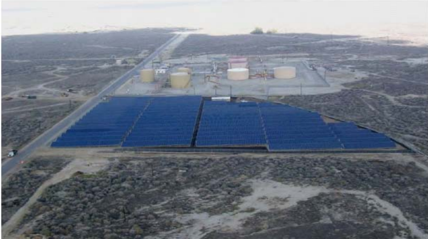
Chevron Solarmine Fellows, CA (near Bakersfield) 614 kWp
