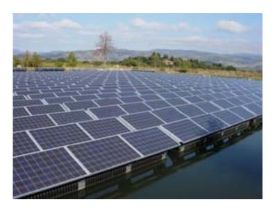
The Floatovoltaic<sup>™</sup> PV System is designed to float on water retention ponds and basins. Uses previously unbuildable space to generate clean, renewable power and mitigates and reduces extensive water-born algae, reducing facility operation and maintenance costs.
