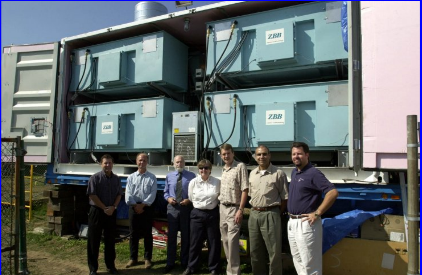
200 kw / 2 hr ZnBr Batteries at Lum, MI Substation
