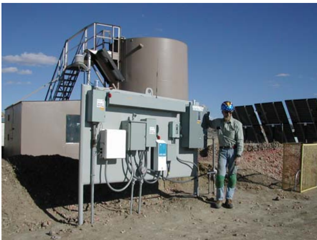
Fig. 1. NREL's Bob Hansen pauses after completing work on a unique, PV powered oil pumping station and data acquisition system at the Rocky Mountain Oilfield Testing Center.
