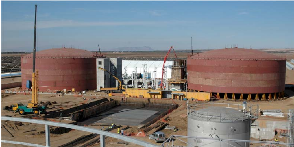
Andasol-1 & 2 plants in Spain: 1,020 MWh, 7.5 full load hrs, 31,000 tons of molten salt
