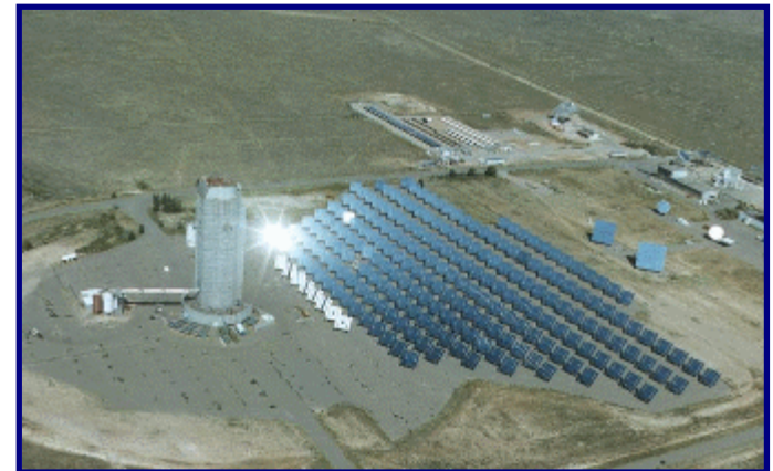
The Solar Power Tower at the NSTTF – 32 years with no upgrades!
