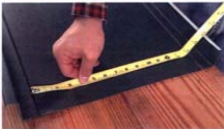
This panel is 16 inches wide, and has a flat surface between ribs. But this panel has shoulder ribs adjacent to each vertical leg, and the width of the flat surface between these shoulder ribs is only 14 inches. Therefore, this profile is also not acceptable for application of the laminate.
