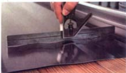
This panel is 18 inches wide, and the surface between the vertical legs does not have stiffener beads of any kind. It does have light striations across the full width of the panel, but these are less than 15 degree angles, and are acceptable. This panel profile also has shoulder ribs, but the distance between the shoulder ribs is approximately 16 inches. Therefore, the laminate can be applied between these ribs.
