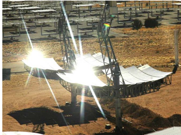
SES Dish Collectors, Sandia National Laboratories, NM
