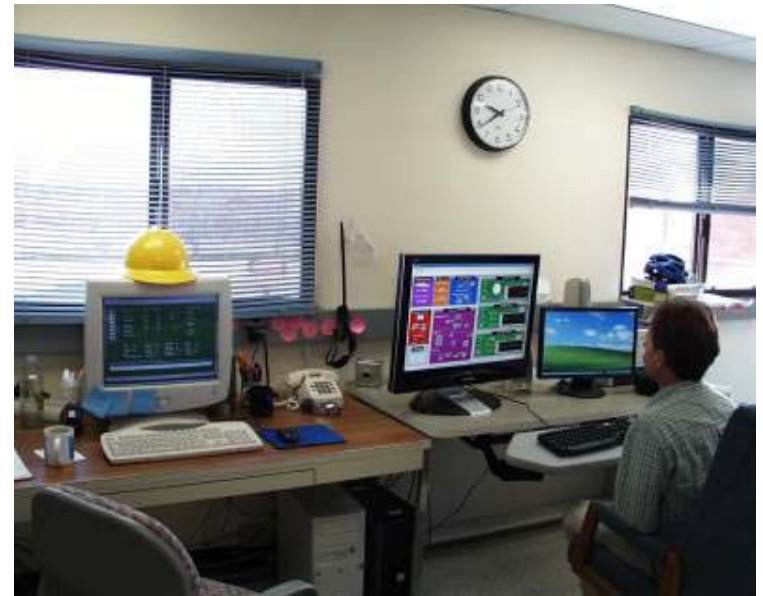
Control room showing tracker and loop controls
