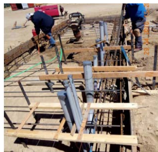
Underground Utilities install
