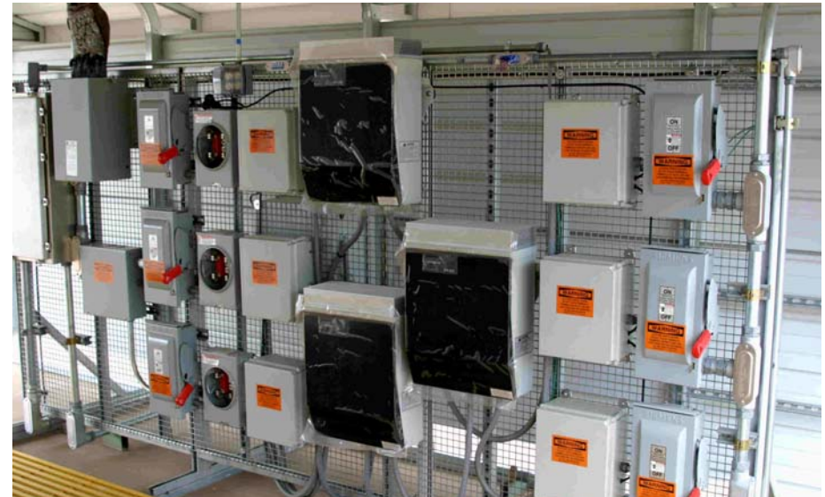
Inverters, combiners, disconnects – all reconfigurable
